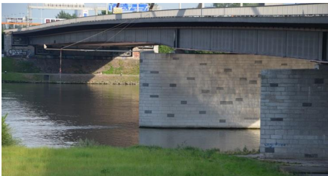
Figure 3: Voest-bridge with existing bridge piers
